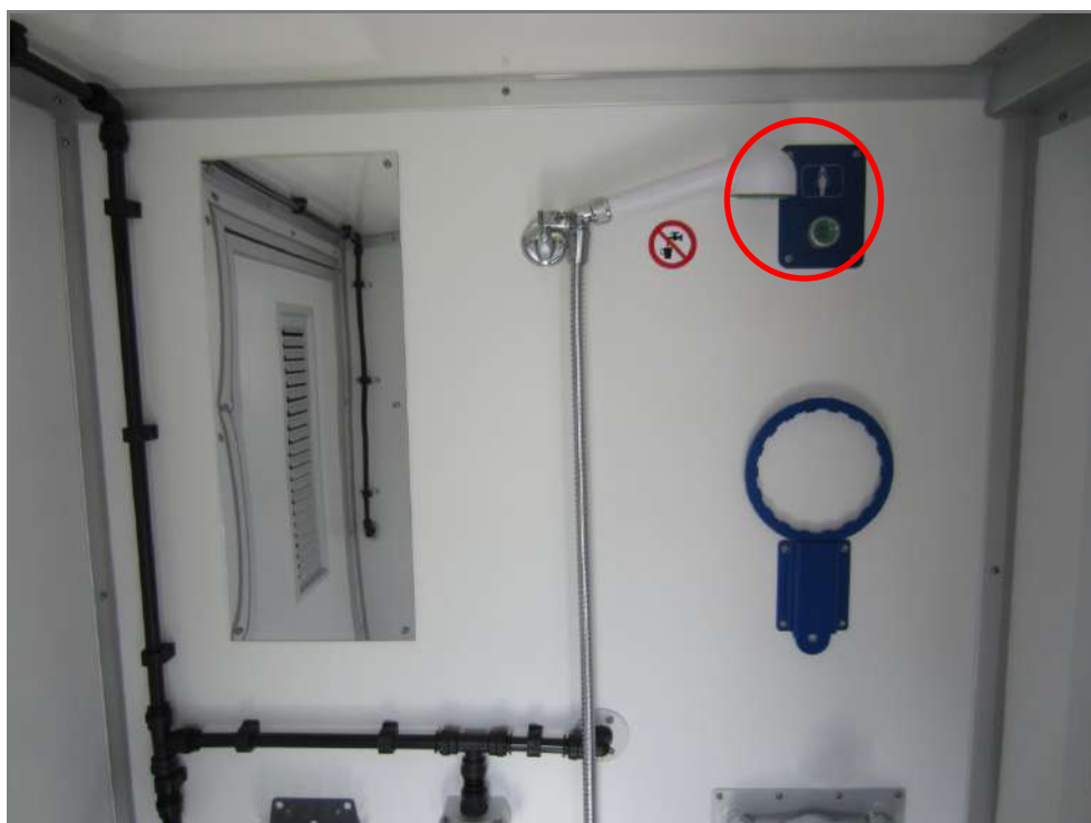
Fig. 1 11 Push-button for activating the shower (red circle)
