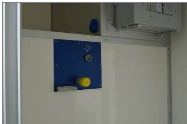
Fig. 1 128 Vacuum cleaner connection
