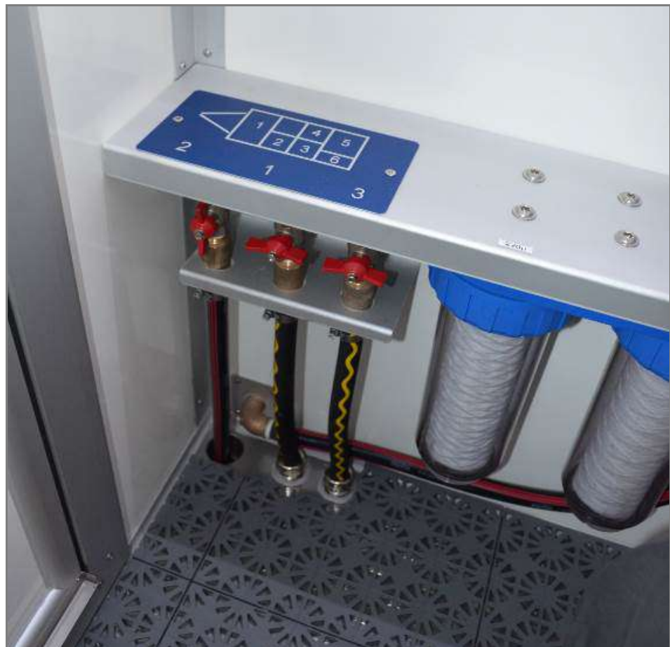
Fig. 1 13 Ball cock in the shower chamber
